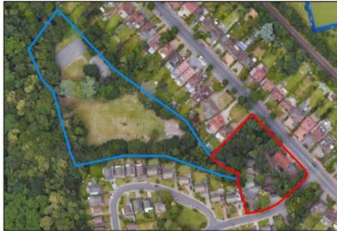
Fig.16 – On-site habitat area in red and off-site habitat area in blue as per BNG assessment (April 2023)
